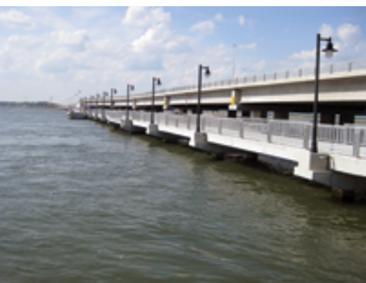
Route 52 Contract A1: The low level bridges with the fishing pier are visible.
