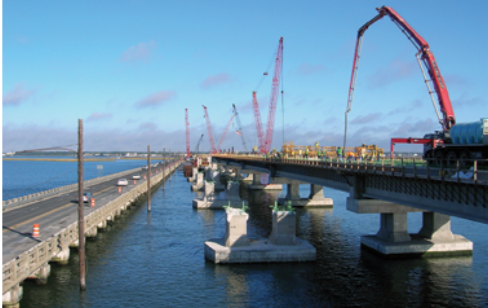
Route 52 Construction of Contract A1, while maintaining traffic on existing causeway.
