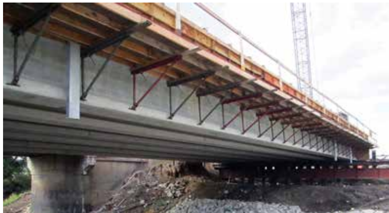
New pretensioned prestressed concrete beam bridge superstructure on temporary supports.
