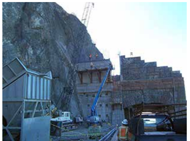
Nearly completed North headwall, looking South.
