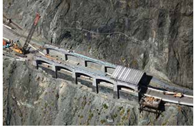
Aerial view of structure with some roof panels in place.
