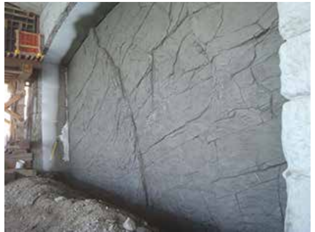
Interior retaining wall architectural treatment, looking Northeast.
