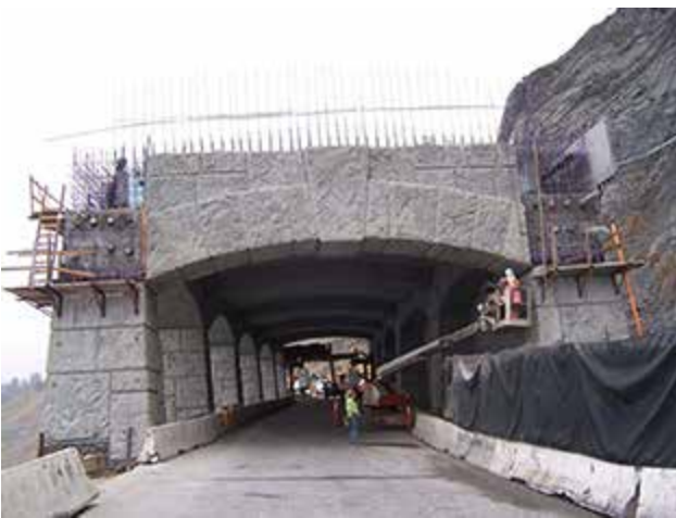
Staged construction of the South headwall, looking North.
