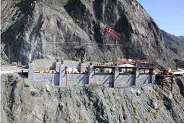
Interior and exterior bents under construction, looking East.
