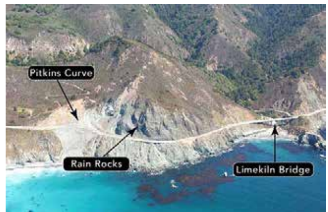
Aerial view looking East of the site before construction.
