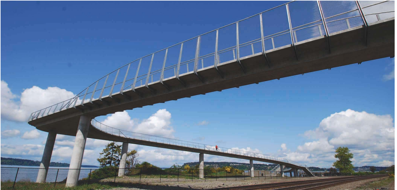
Underside view of the 106-ft-long span over the railroad tracks. The 30-ft-wide viewing platform is at the left edge of the photo and the stairs to the beach are to the right. All photos: BergerABAM.
