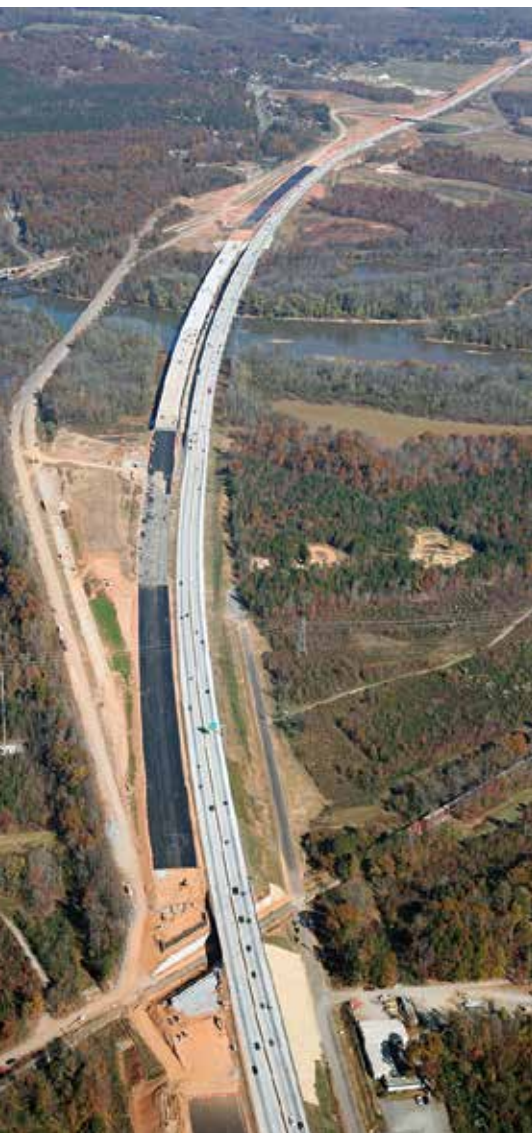
Northbound bridge opened early to improve safety. Photo: STV.
