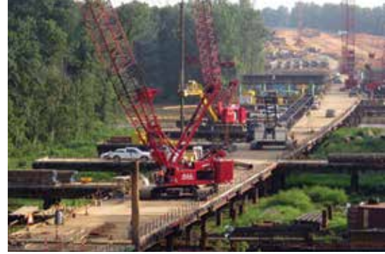
The 2500-ft-long work trestle. Photo: STV.
