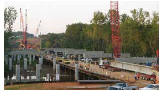
Girder delivery at the southern end of the bridges. Photo: Flatiron.
