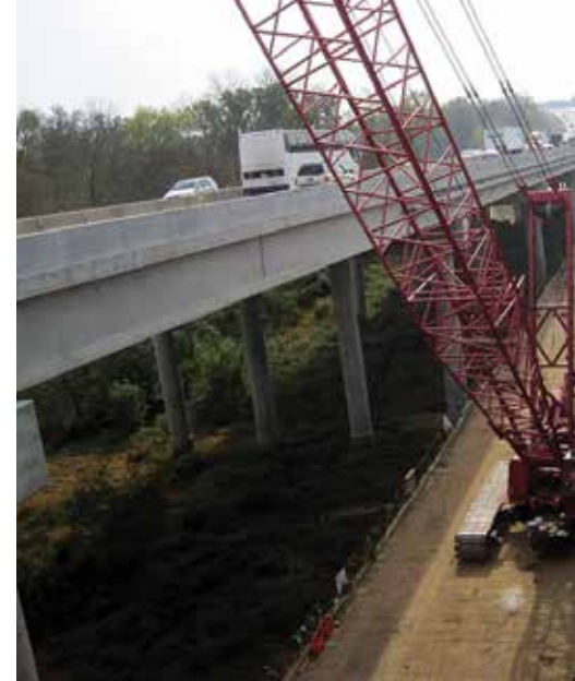
North end of the work trestle. Photo: STV.
