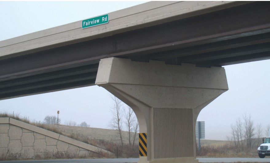
Figure 9. Fairview Road Bridge over Interstate 80, near Omaha, Neb., utilizing continuous-for-live load details. Photo: e.construct.USA.
