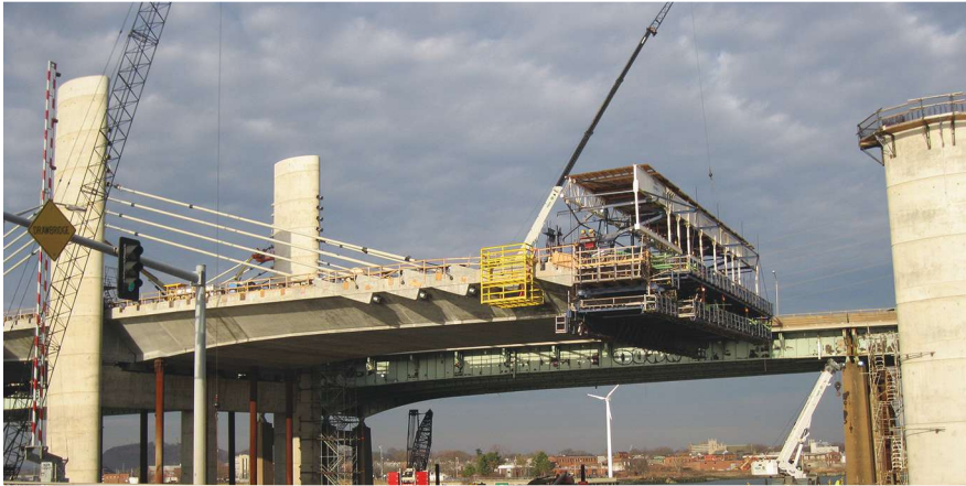
Cantilever construction on the northbound bridge. Photo: AECOM.
