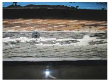
Corroded strands in a bonded post-tensioning tendon.
