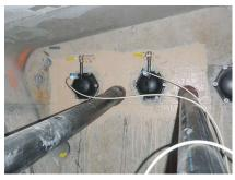
Impregnation of post-tensioning tendon from end anchorage.
