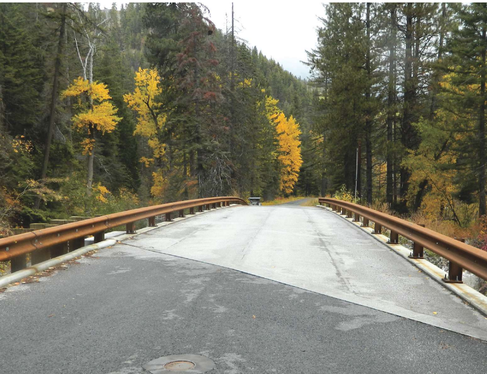
Finished deck of skewed decked bulb-tee girders for the Old Blewett No. 1 Bridge, Chelan County, Wash. Photo: Chelan County Public Works Department.
