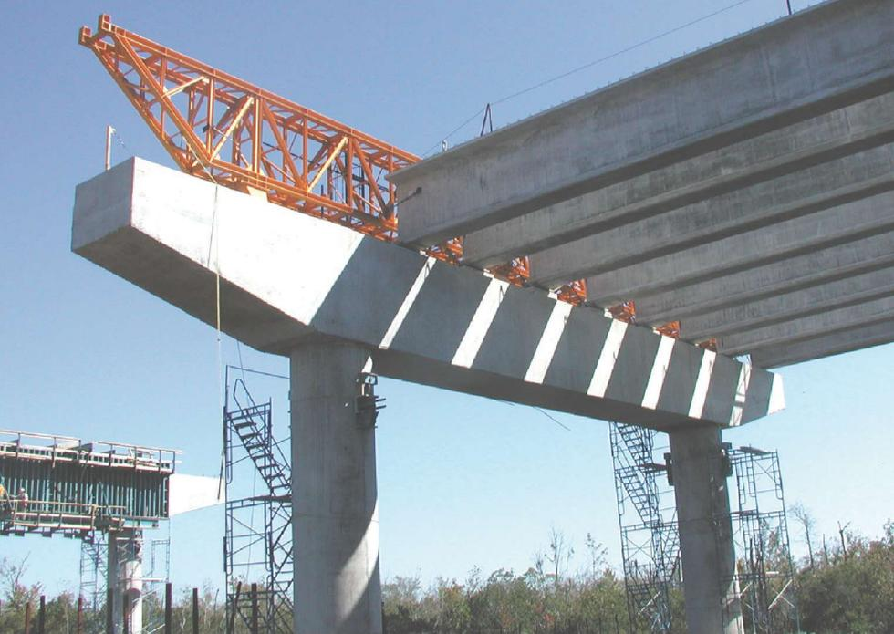
Fifty-seven spans on the Interstate 45 Galveston Causeway bridge feature 72-in.-deep prestressed concrete girders. The frame on the pier cap is part of a system for erecting the girders. Photo: Traylor Bros. Inc.
