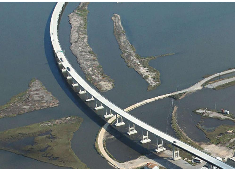
The Louisiana Highway LA1 relocation project Phase 1B has a 4-mile-long, high-level bridge featuring prestressed concrete piles, cast-in-place substructures, Type III and BT-78 prestressed concrete girders, precast concrete deck panels, and a cast-in-place concrete deck. Photo: Traylor Bros. Inc.
