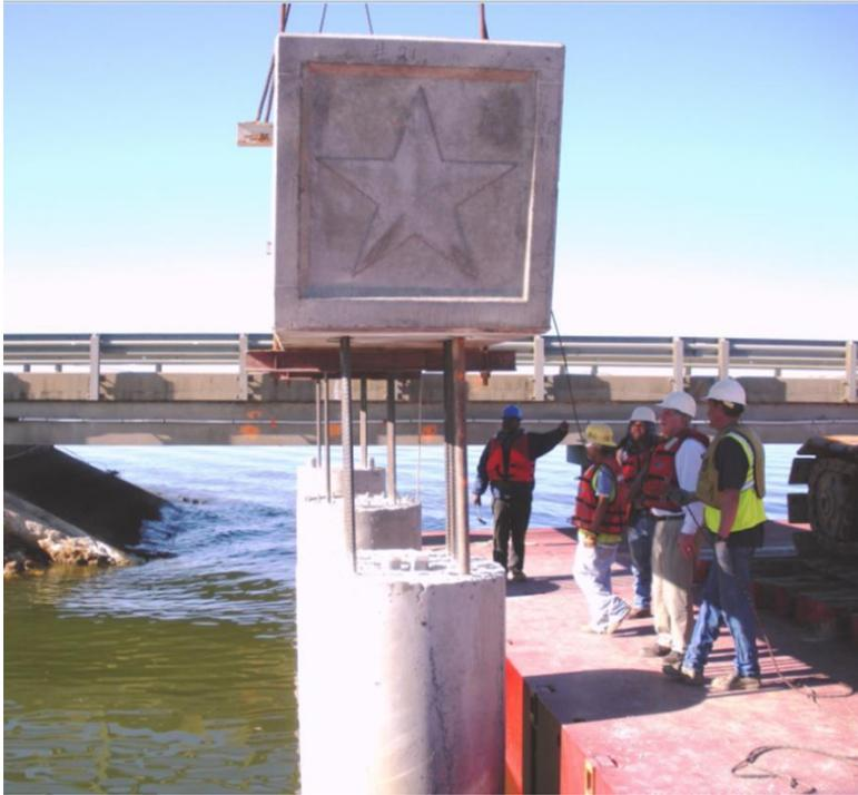
Prior to casting cap, top and bottom of corrugated steel pipe must be sealed off with round removable forming plugs. Remove plugs prior to placing cap on columns.
