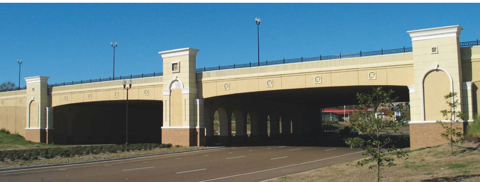
The U.S. Highway 61/84 Bridge over Liberty Road in Natchez, Miss., presents examples of precast concrete aesthetic panels and castings that the Mississippi Department of Transportation is able to add to bridges at a lower cost with a robust concrete industry in Mississippi.
