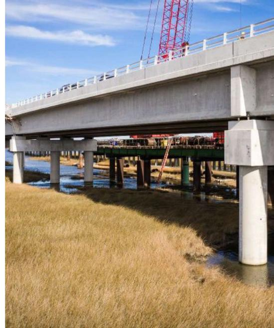
The use of precast concrete pile bents and vertical cylinder pile foundations minimizes the project's permanent impact on environmentally sensitive seagrass beds in the north approach spans.
