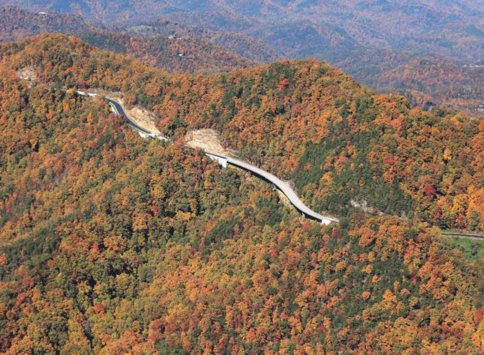
Aerial view of the "Missing Link." Bridge 2 is visible in the center. Photo: Eastern Federal Lands Highway Division of the Federal Highway Administration.
