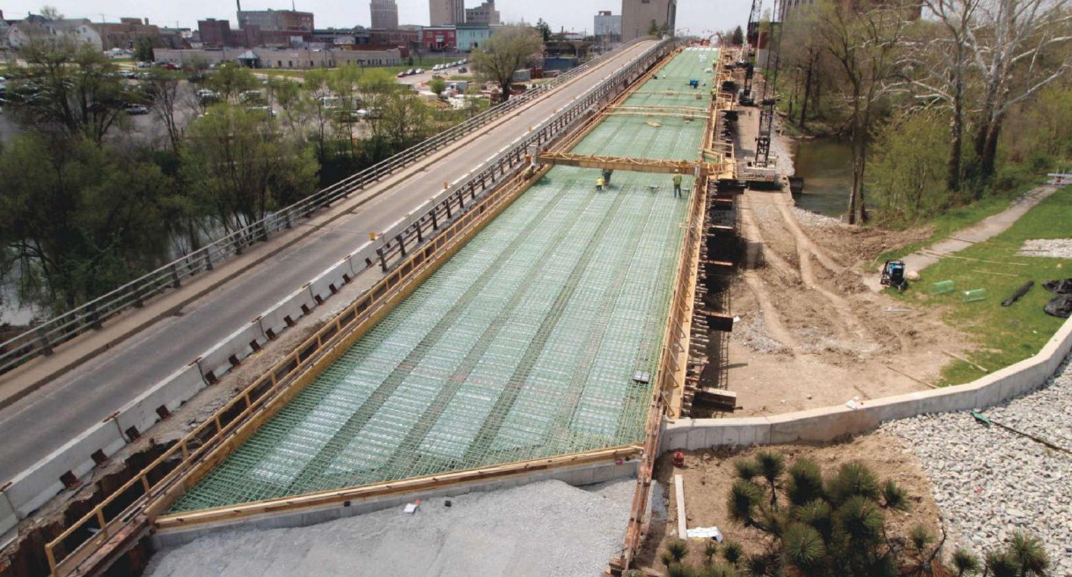
Epoxy-coated reinforcement was used in the 8-in.-thick deck. Photo: United Consulting.
