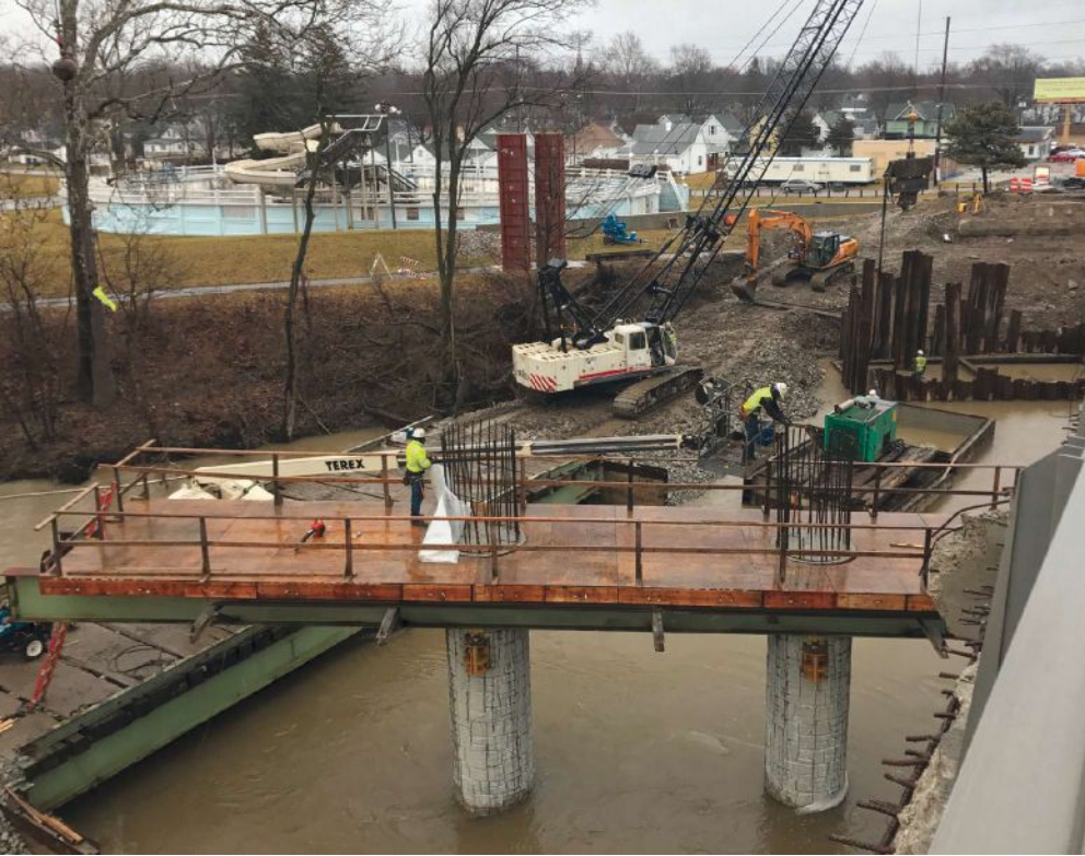
Pier cap and footing construction. Photo: United Consulting.
