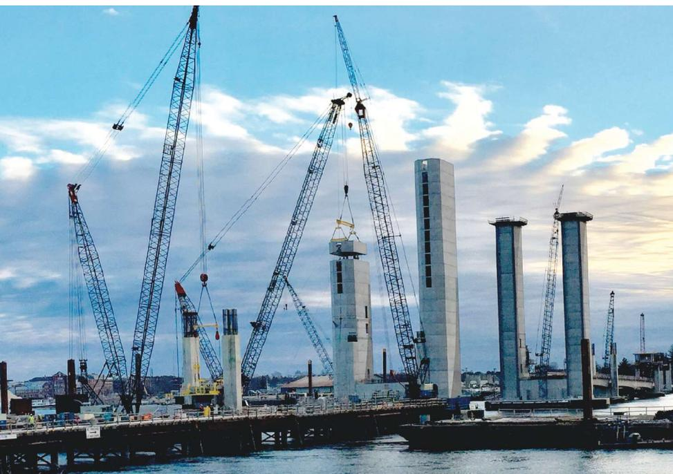
Each lift tower consists of 21 precast concrete segments cast at the project site using match-casting procedures. Photo: Maine Department of Transportation.
