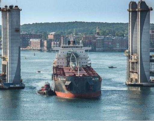
A ship passing through the movable span during construction shows the added width for maritime traffic and the size of ship that needs to be accommodated. Photo: Maine Department of Transportation.
