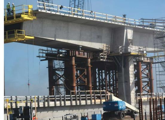
The upper vehicular spans feature precast concrete segmental box girders with depths varying between 8 and 13.5 ft and base widths varying from 15 to 16.75 ft. Photo: Maine Department of Transportation.
