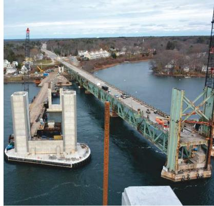
A new alignment was created for the replacement bridge, reducing the crossing skew to 15 degrees for approaching ships. Photo: Maine Department of Transportation.
