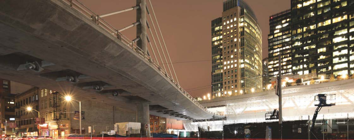
The bus ramp cable-stayed bridge at night with box girders, link beams, and stay anchorages visible. Photo: Arup.
