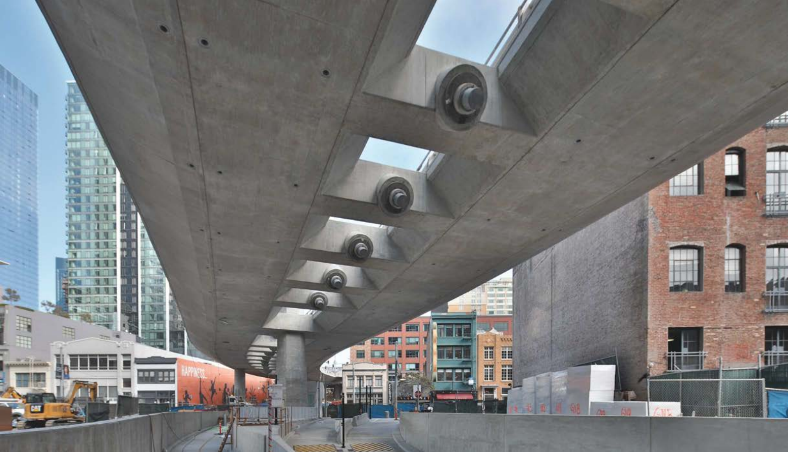
Underside of the bridge showing box girders, link beams, and stay anchorages. Photo: Arup.
