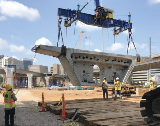
The erection of a split-pier segment. Photo: Structural Technologies.
