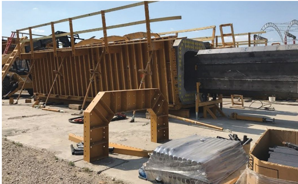
Precast concrete column in form with core form being extracted. Photo: Johnson Bros.
