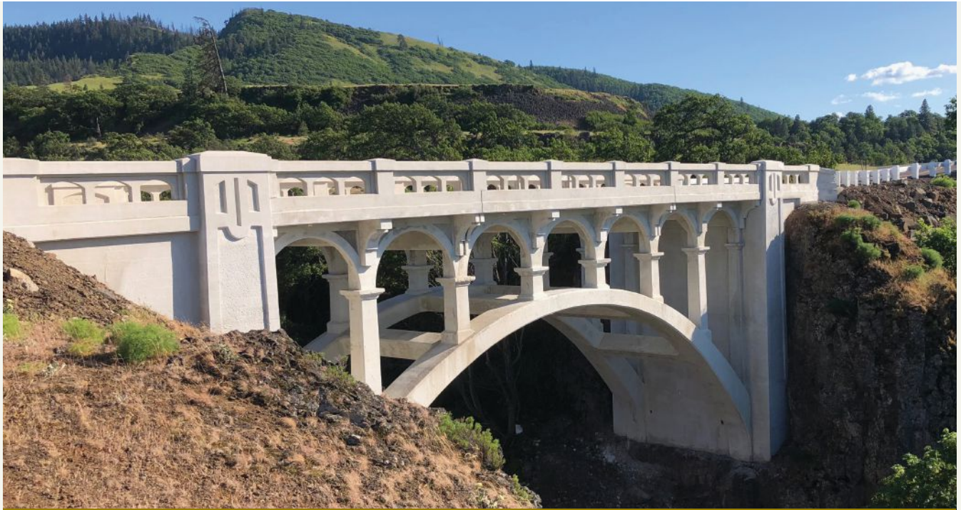
After being coated with a cementitious render and silane sealer, the rehabilitated bridge looks almost brand new. Photo: Rebecca Burrow.
