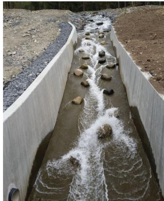
Because debris and water flows are expected to increase as the climate changes, Norway has installed debris deflectors or screens on newer projects (top) to keep debris out of drainage systems, and energy dissipaters in channels and culverts (bottom) to reduce velocities.
