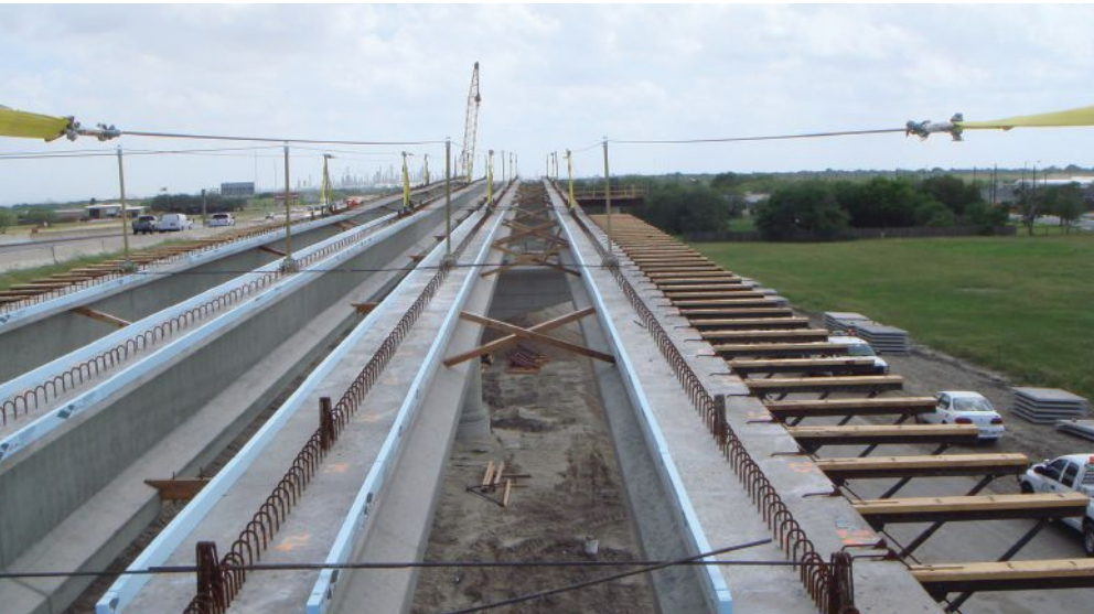
Figure 3. Timber X-bracing (left) was a required element in previous bracing standards for the Texas Department of Transportation (TxDOT). However, this bracing would sometimes lose contact with the girder due to fascia beam rotation during deck construction (right). The new TxDOT standard bracing detail uses horizontal timber bracing between the bottom flanges.
