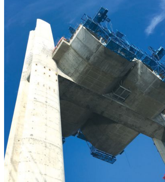
Figure 1. At the St. Croix Crossing in Oak Park Heights, Minn., a cast-in-place pier cross beam interfaces with a precast concrete segmental box-girder superstructure. In some cases, both the cast-in-place element and the precast concrete segment can satisfy their own dimensional tolerances but not match each other. All Photos: McNary Bergeron & Associates.
