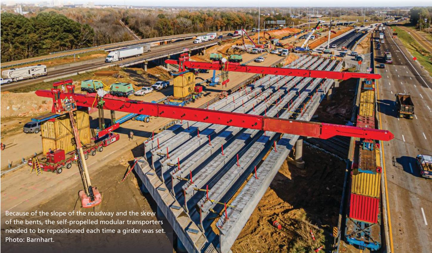
Because of the slope of the roadway and the skew of the bents, the self-propelled modular transporters needed to be repositioned each time a girder was set. Photo: Barnhart.
