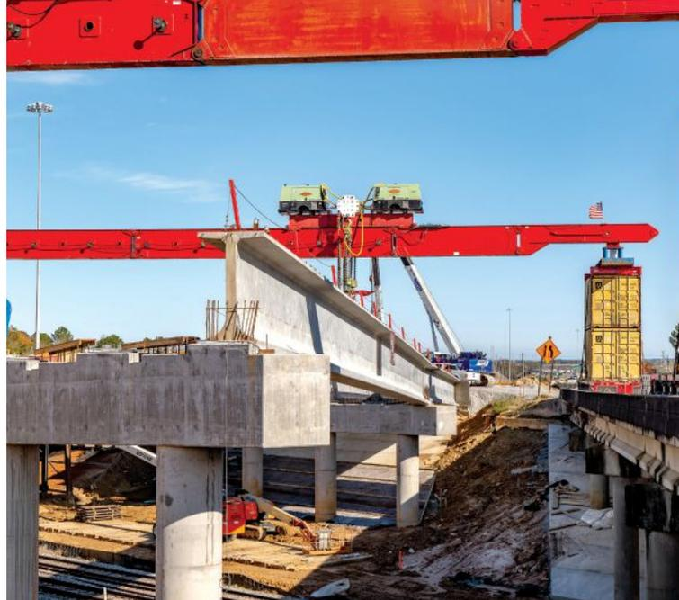
The first 170-ft-long, 200,000 lb girder after it was erected over the railroad. Photo: Key Constructors.
