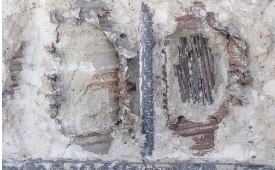
Deck tendon after excavation and opening of ducts for inspection.
