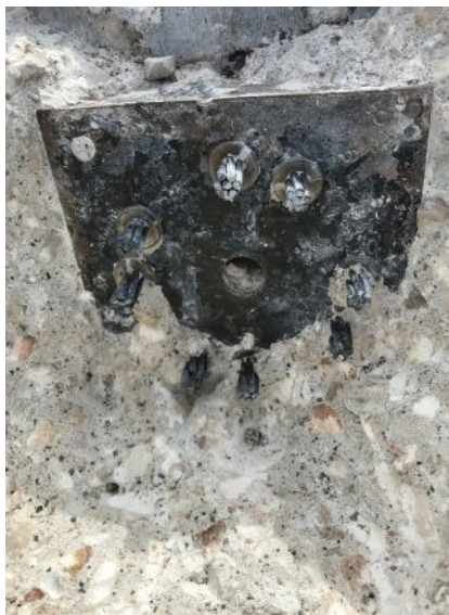
Continuity tendon anchor in deck exposed for inspection.
