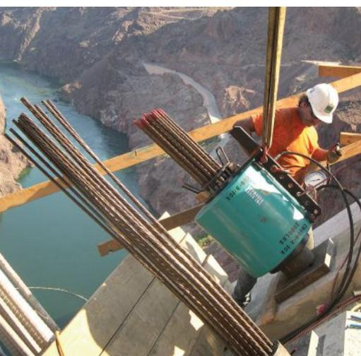
On the Hoover Dam Bypass Bridge, one of the largest concrete arch bridges in the world, Schwager Davis supplied the temporary stay-cable system and post-tensioning materials for this iconic bridge's twin arches that meet at midspan over the Colorado River. The firm's crews worked post-tensioning two temporary towers on both sides of the bridge. The peak of these towers served as the location for cables to be attached.
