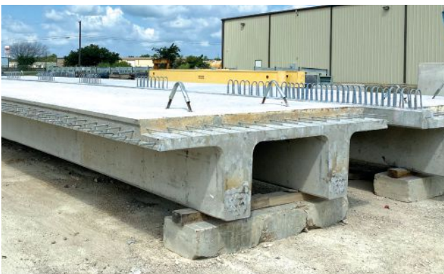
NEXT D beams stored at the precaster's plant. The top and bottom transverse reinforcement project from the sides of the top flange for the ultra-high-performance concrete closure pour. The top and bottom bars are staggered to avoid conflicts during erection. The notch in the top flange at the end of the beam is for a closure pour to make the flange continuous and avoid an open joint.
