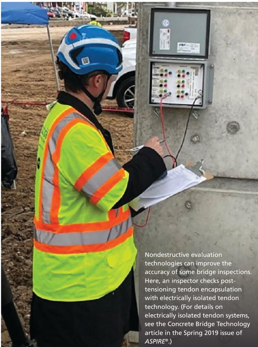
Nondestructive evaluation technologies can improve the accuracy of some bridge inspections. Here, an inspector checks post-tensioning tendon encapsulation with electrically isolated tendon technology. (For details on electrically isolated tendon systems, see the Concrete Bridge Technology article in the Spring 2019 issue of *ASPIRE*®.)
