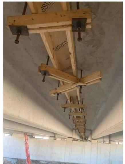
Formwork for the ultra-high-performance concrete (UHPC) closure pours between NEXT D beams. This was the second project in Texas to use UHPC.
