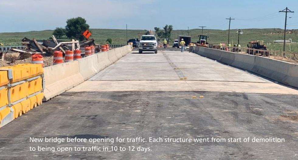
New bridge before opening for traffic. Each structure went from start of demolition to being open to traffic in 10 to 12 days.
