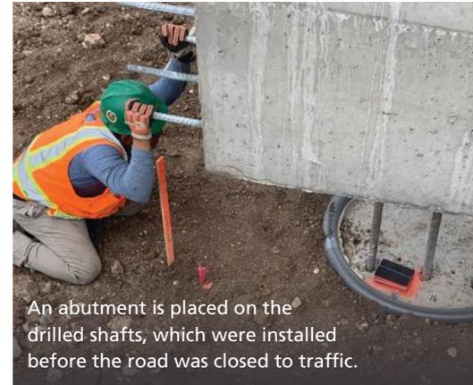
An abutment is placed on the drilled shafts, which were installed before the road was closed to traffic.
