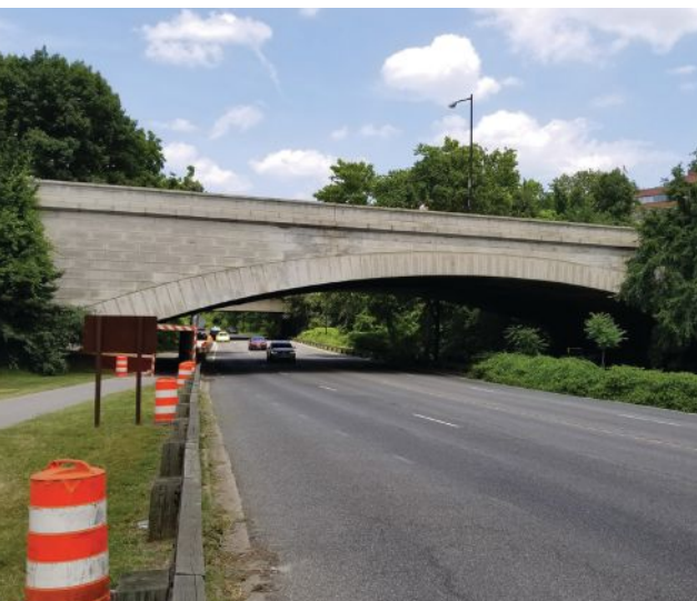
Pennsylvania Avenue Bridge over Rock Creek Parkway. Originally constructed in 1858 of 48-in.-diameter cast iron water mains as the load-bearing arch members, the bridge was one of the largest single-span iron pipe arch structures in the world. In 1913 a concrete arch bridge was constructed around the original bridge. The concrete superstructure was reconstructed in 1979, and the arch and superstructure were rehabilitated in 2018 to extend the bridge's service life. Photos: District Department of Transportation.
