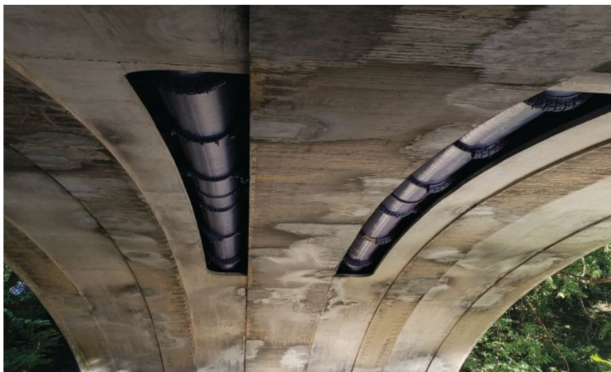
Pennsylvania Avenue Bridge over Rock Creek Parkway. Originally constructed in 1858 of 48-in.-diameter cast iron water mains as the load-bearing arch members, the bridge was one of the largest single-span iron pipe arch structures in the world. In 1913 a concrete arch bridge was constructed around the original bridge. The concrete superstructure was reconstructed in 1979, and the arch and superstructure were rehabilitated in 2018 to extend the bridge's service life. Photos: District Department of Transportation.
