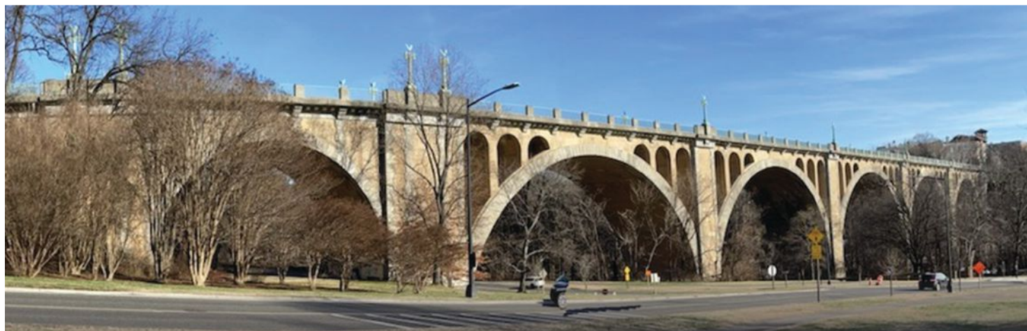
William Howard Taft Bridge, which carries four lanes of Connecticut Avenue traffic over Rock Creek, Beach Drive, and Cathedral Avenue, is an 1841-ft-long, five-span, unreinforced concrete, open- and closed-spandrel arch structure with a reinforced concrete deck. Completed in 1907, it was one of the first and largest unreinforced concrete bridges in the world. Photo: District Department of Transportation.
