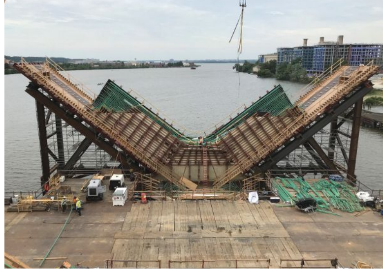
Each V-pier of the Frederick Douglass Memorial Bridge required 950 yd 3 of concrete, completed in four mass placements with cooling tubes. Photo: District Department of Transportation and HNTB.
