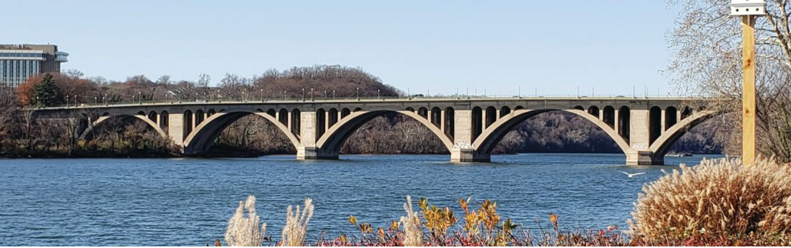
The Francis Scott Key Bridge crossing the Potomac River is a reinforced concrete open-spandrel, ribbed-arch bridge, which was completed in 1923. Designed in the Classical Revival style by Nathan C. Wyeth, the bridge was added to the National Register of Historic Places in 1996. Photo: District Department of Transportation.
