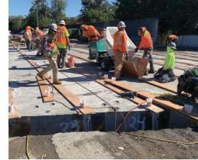
As each successive joint was filled with ultra-high-performance concrete, secondary crews installed cover plates, positive head-pressure ports, and temperature-monitoring embeds.
