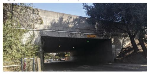
Originally constructed in 1959, the 21st Avenue undercrossing on State Route 99 is the primary vehicle and pedestrian route linking the Oak Ridge and North City Farms neighborhoods of Sacramento, Calif. Although the abutments and substructure were sound, delamination of a previous overlay, soffit cracking, and other deterioration led to the decision to replace the superstructure. All Photos: California Department of Transportation.
