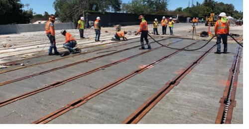
Immediately following installation of the box beams, crews installed joint caps and seals and performed the required surface saturation and leak testing before placing ultrahigh-performance concrete in the joints.
