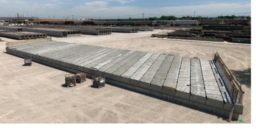
Preassembly of the completed beams at the precaster's facility allowed verification of cumulative casting tolerances and fit-up.
