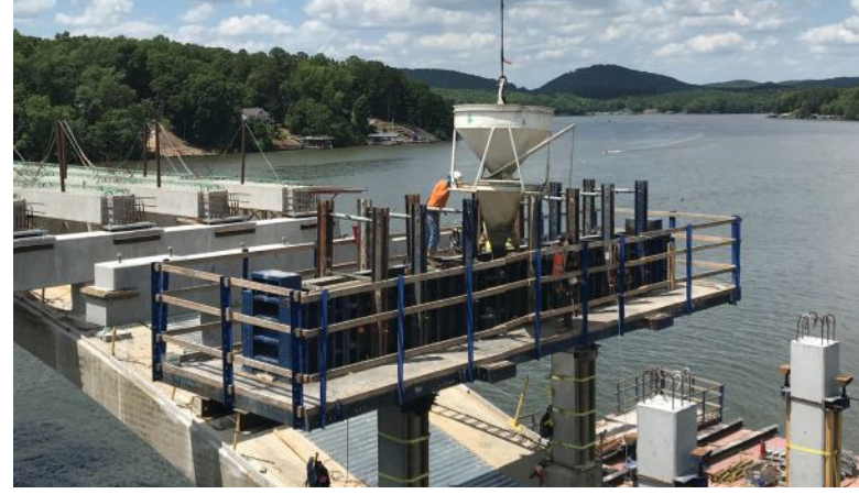
Cast-in-place concrete cap construction.
