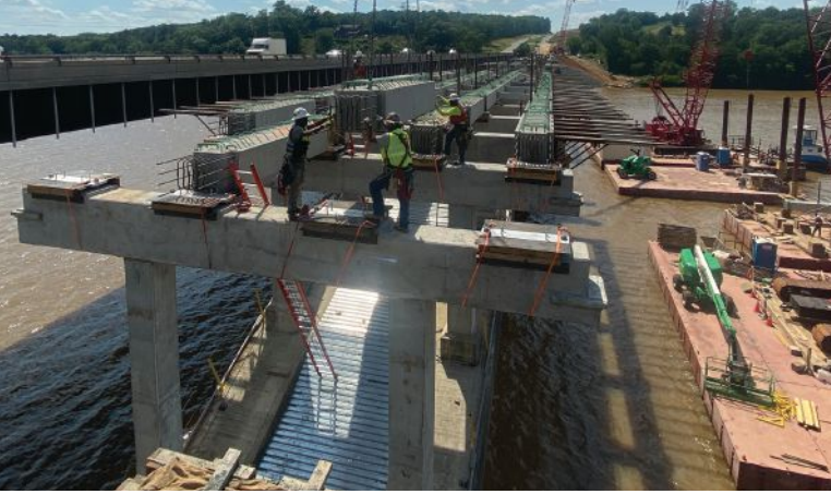
New precast concrete box beams are erected in span F. Note the continuity reinforcement detail at the beam end, the common bearing under the continuity diaphragm, and the epoxy-coated reinforcement that will be cast into the composite deck.
