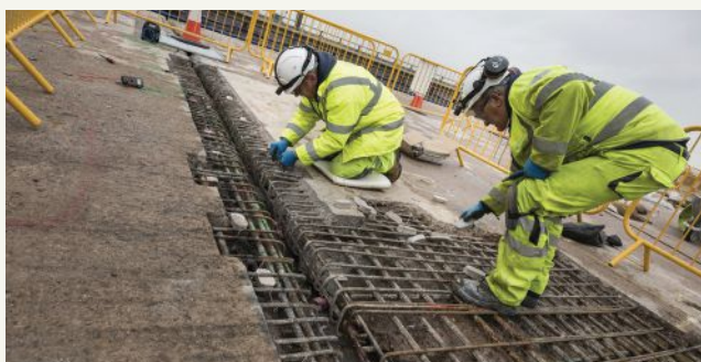
Figure 4. Type 1 galvanic anodes are placed in a concrete repair area to prevent future reinforcing steel deterioration and extend the service life of the repair. Photo: Vector Corrosion Technologies.
