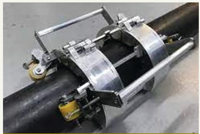
Magnetic flux leakage technology being used on an external tendon to detect section loss and wire breaks in post-tensioning strands. Photo: Infrastructure Preservation Corporation.
