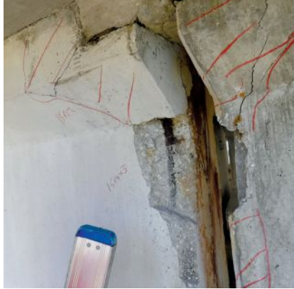
Cracks and spalls being measured and documented during a bridge inspection.
