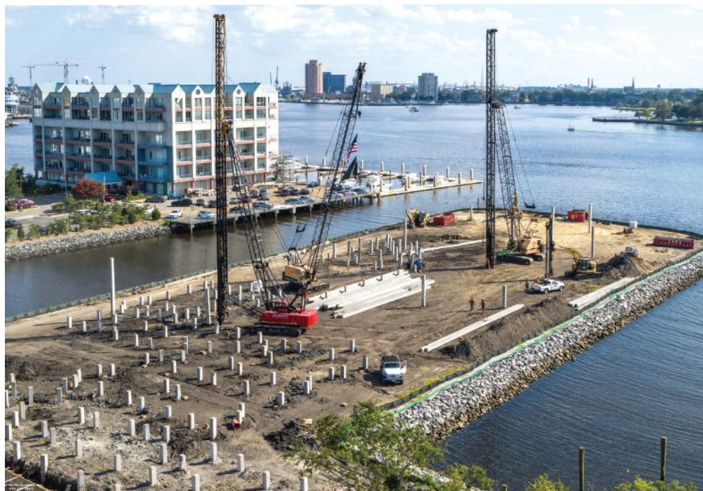
A typical on-land pile-driving operation allows piles to be stockpiled on site for easy access. Precast, prestressed concrete piles are displacement piles that create no spoil at the site. Photo: Concrete Technology Corp.
