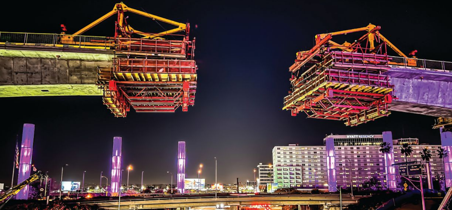
Nighttime view of form travelers being used during concrete segmental construction of the 212-ft span over Sepulveda Boulevard. Photo: Los Angeles World Airports.
