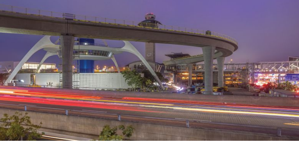
The guideway under construction in front of the iconic Los Angeles International Airport theme building. Note the expansion joint visible in the guideway at the pier. Photo: HDR Inc.
