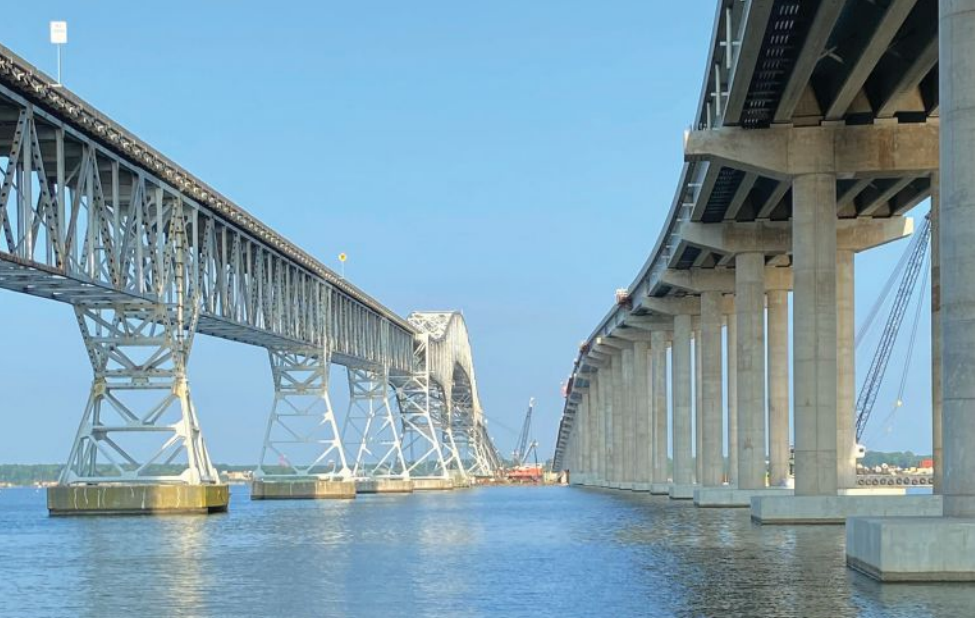
The new concrete bridge (right), designed for a 100-year service life, will be more durable and require less maintenance than the previous steel structure (left). Photo: AECOM.
