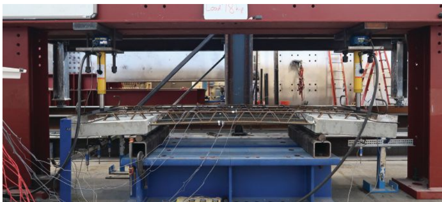
Figure 4. The NextGen bridge deck research project, which is being conducted at University of Texas at Austin, is studying partial-depth precast concrete deck panels. Results of this research project, as well as other projects involving bridge deck construction, will be incorporated into the Bridge Deck Construction Inspection Program.
