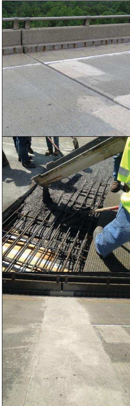
Figure 4. Before, during, and after photos of eliminating a joint on an existing bridge. This intervention is commonly used in the bridge preservation program in Virginia. Jointless construction is required for new bridges in Virginia.
