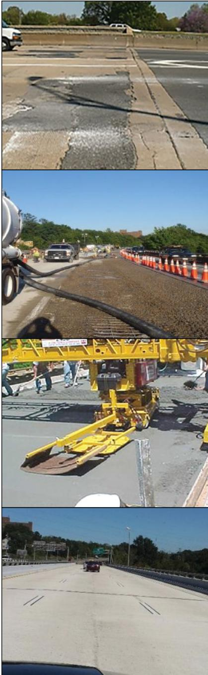
Figure 3. The use of latex-modified and silica fume concrete for overlays, in conjunction with hydromilling, extends the service life of a bridge by three to four decades. It is a mainstay of Virginia's bridge preservation program.
