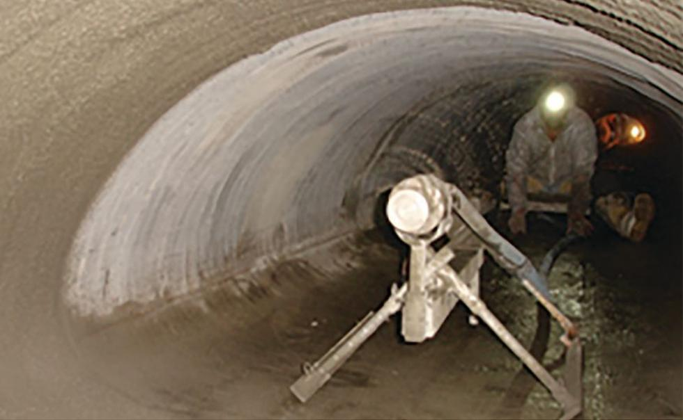
Figure 6. A spray-on liner using fiber-reinforced concrete is installed to extend the service life of a steel culvert structure.
