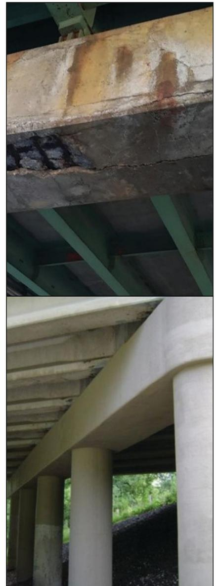
Figure 5. Examples of substructure deterioration (top) and a substructure repaired by localized hydromilling and repair with self-consolidating concrete followed by the application of a coating (bottom).
