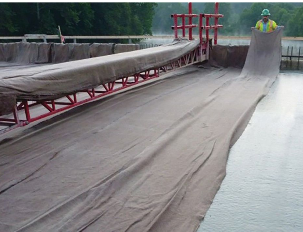
Figure 2. Wet burlap is placed immediately after screeding.
