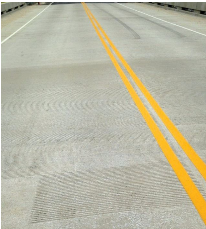
Figure 1. Bridge decks using low-shrinkage concretes with no cracks after one year of exposure. The bridge deck on the left was constructed with normalweight concrete, and the bridge deck on the right used lightweight concrete. All Figures: Virginia Department of Transportation.
