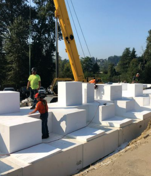
At the roadway approaches, geofabric blocks are placed over traditional gravel materials to mitigate settlement of the highly compressible peat layers. Photo: City of Kenmore.
