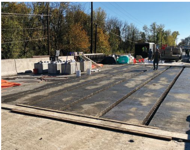
Figure 3. Precast, prestressed concrete slabs for the West Fork Dairy Creek Bridge after erection. The joints were soaked with water to create a saturated surface-dry condition, and concrete ecology blocks were used for adjusting differential camber.
