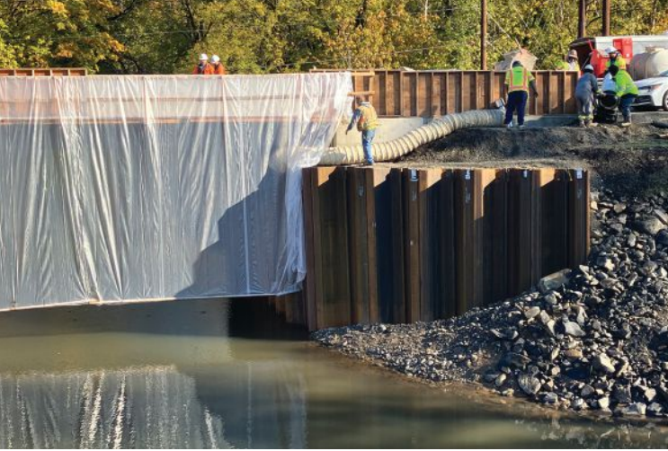
Figure 5. Heating with containment is used for cold-temperature mitigation during the ultra-high-performance concrete closure pours.
