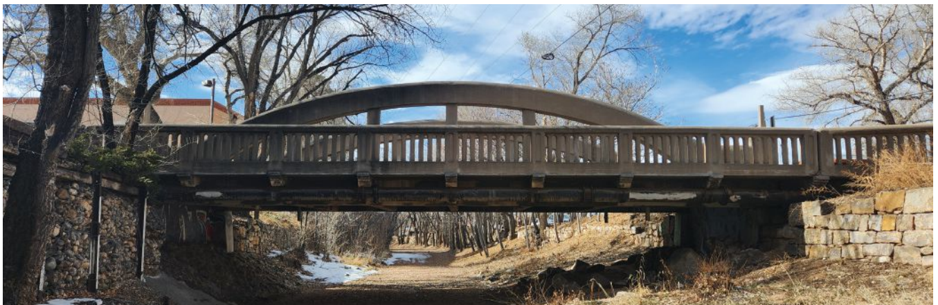
Figure 2. One of New Mexico's oldest bridges carries Grant Avenue over Arroyo de Las Mascaras in the heart of Santa Fe. The concrete through-truss bridge, dubbed the "Rainbow Bridge," was built in 1920. Photo: New Mexico Department of Transportation.
