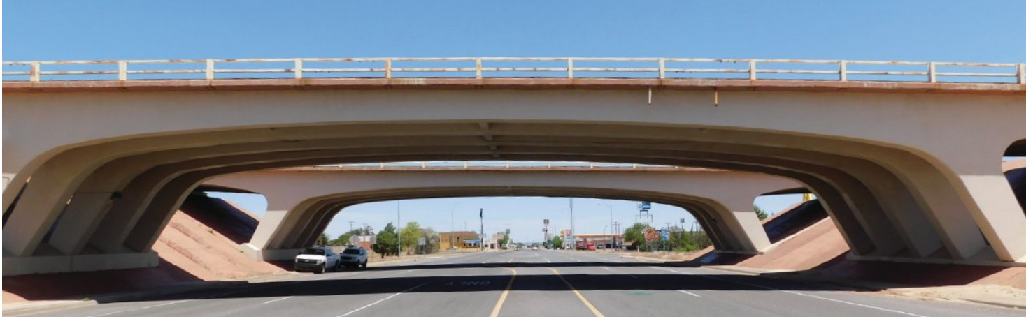
Figure 3. Two of the New Mexico Department of Transportation's concrete K-frame bridges carry Interstate 40 in Tucumcari, N.Mex. There are eight K-frame bridges in the state. Photo: New Mexico Department of Transportation.
