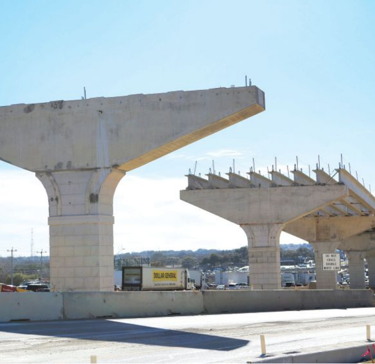
On the Interstate 35 Northeast Expansion Central Project in the San Antonio, Tex., area, Consor was responsible for the design of 7.6 miles of elevated structures, which included more than 350 prestressed concrete hammerhead bent caps on top of cast-in-place columns. The left photo shows prestressed concrete girders on prestressed concrete hammerhead bent caps, and the right photo shows the architectural details of the cast-in-place columns and the protruding reinforcement for the connection to the precast concrete bent caps. Photos: Alamo NEX Construction.
