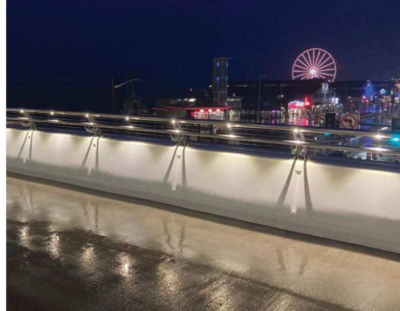
View from the top of the main-span bridge showing the stainless steel railing, pod lights, and a scenic view of the Seattle Waterfront.
