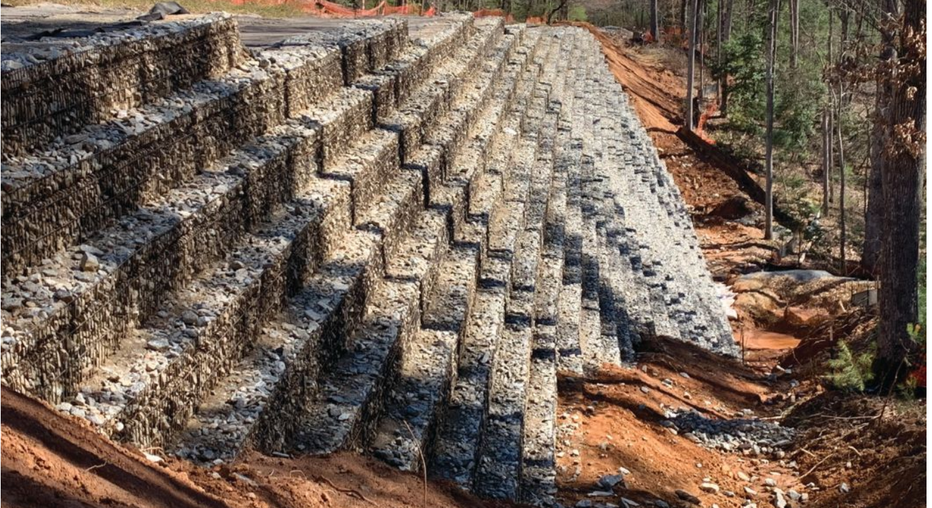
The reinforced-soil retaining wall at the Abutment 2 approach will have native grasses growing on the gabion baskets.
