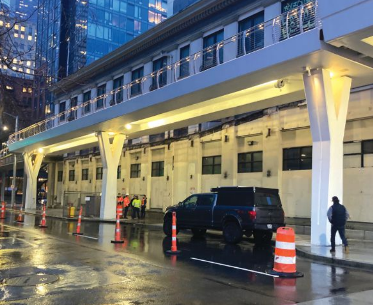
The two-span approach bridge, a cast-in-place, post-tensioned concrete slab structure, connects to the east cantilever of the main-span bridge.
