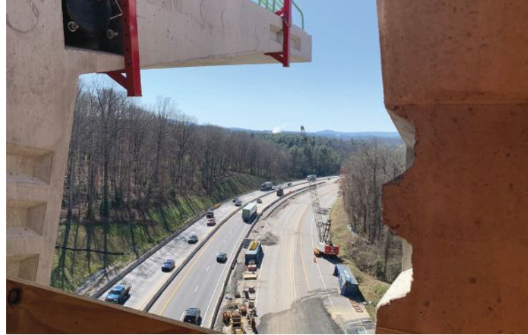
View of Interstate 26 through the main-span closure pour opening. The shear keys on the precast concrete segments are visible on the left and right sides of the photo.
