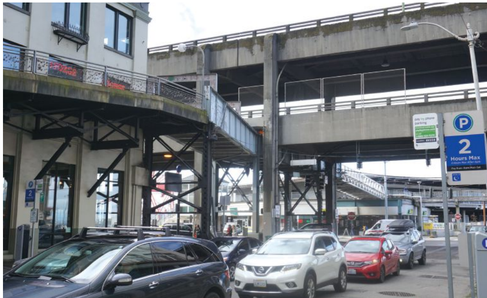
Photo from 2019 showing the previous pedestrian structures, which included a section that traveled beneath the State Route 99 (Alaskan Way) viaduct. The double-deck viaduct has since been demolished and replaced with a tunnel.
