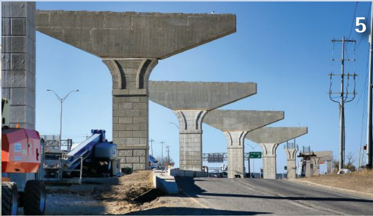
Photo: Alamo NEX Construction.
