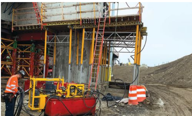
The approximately 93-ft-long straddle bent used 14 longitudinal post-tensioning tendons—each with nineteen 0.6-in.-diameter strands—within the 9 ft × 9 ft cross section.
