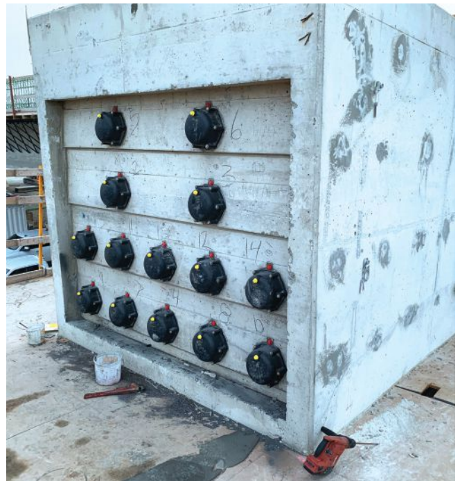
The approximately 93-ft-long straddle bent used 14 longitudinal post-tensioning tendons—each with nineteen 0.6-in.-diameter strands—within the 9 ft × 9 ft cross section.
