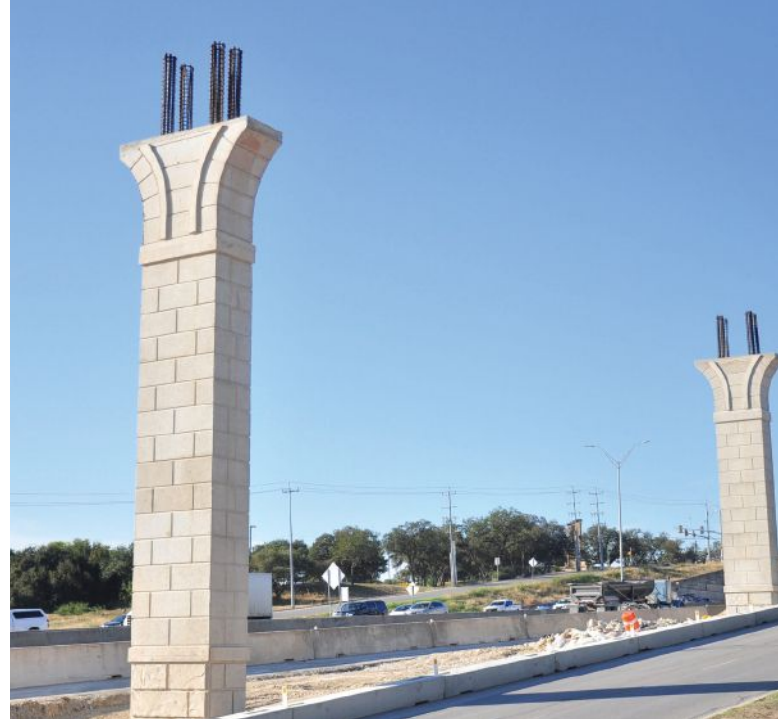
On the Interstate 35 Northeast Expansion Central Project in the San Antonio, Tex., area, Consor was responsible for the design of 7.6 miles of elevated structures, which included more than 350 prestressed concrete hammerhead bent caps on top of cast-in-place columns. The left photo shows prestressed concrete girders on prestressed concrete hammerhead bent caps, and the right photo shows the architectural details of the cast-in-place columns and the protruding reinforcement for the connection to the precast concrete bent caps. Photos: Alamo NEX Construction.
