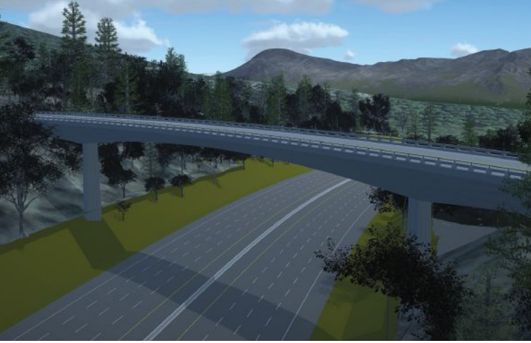
Rendering of the three-span Blue Ridge Parkway bridge over Interstate 26 with the Blue Ridge Mountains in the background.
