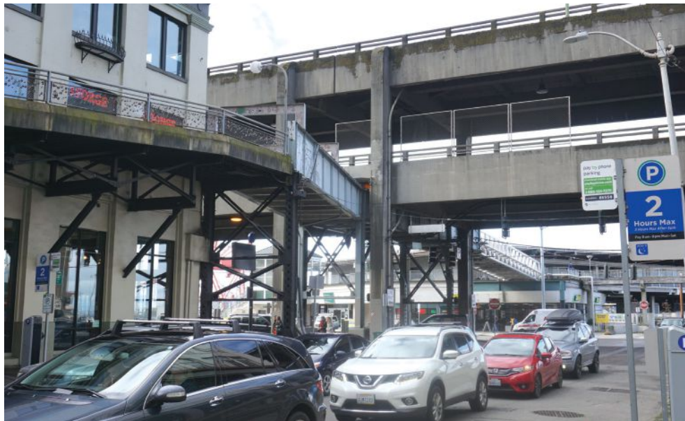
Photo from 2019 showing the previous pedestrian structures, which included a section that traveled beneath the State Route 99 (Alaskan Way) viaduct. The double-deck viaduct has since been demolished and replaced with a tunnel.
