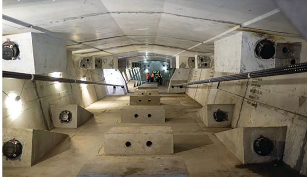
View inside the Laurel Fork Bridge showing the external epoxy-coated-strand tendons. Workshop participants were able to walk through the inside of the bridge and view the hardware and details of the unducted post-tensioning system. Photo: Gregg Freeby, American Segmental Bridge Institute.
