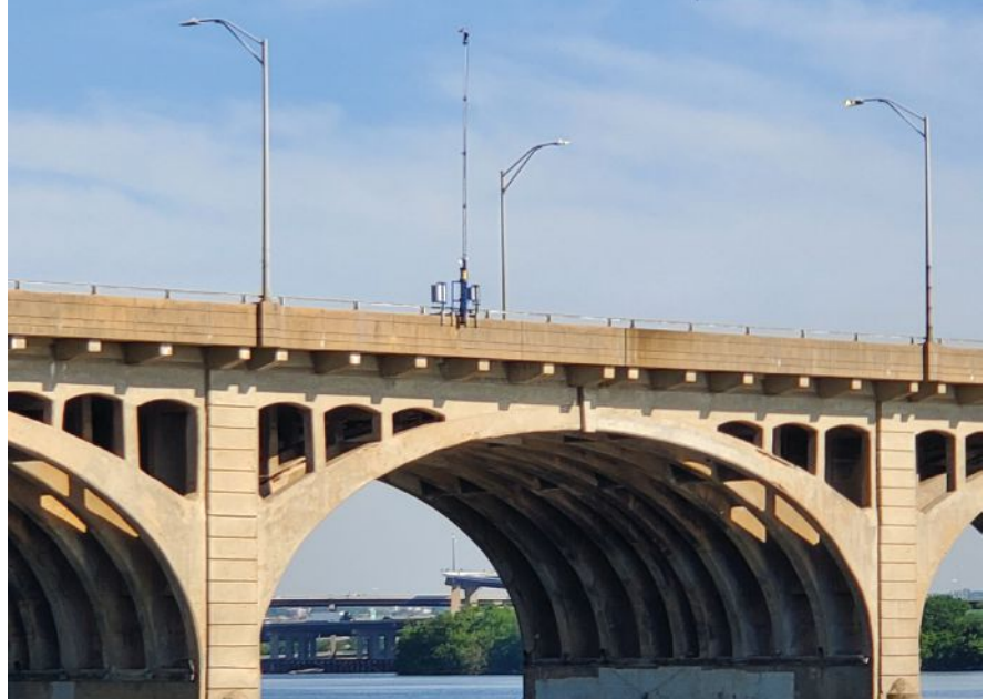
On the Hanover Street Bridge (Vietnam Veterans Memorial Bridge) in Baltimore, Md., infrared ultra-time domain measurements were taken to assess subsurface defects in the concrete deck. All Photos: Fuchs Consulting Inc.
