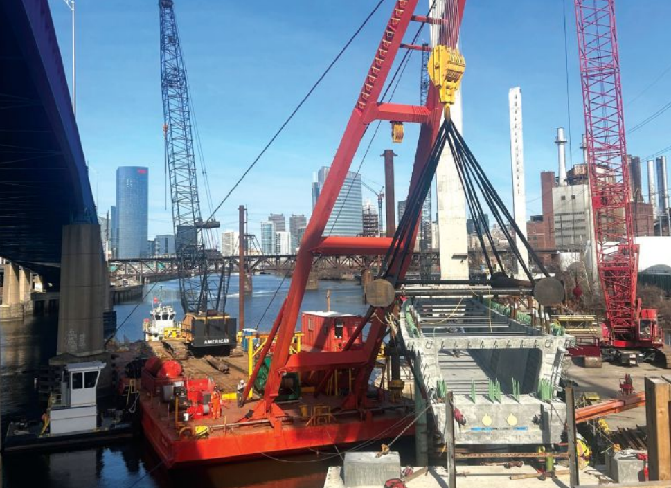
Barge-mounted crawler assist crane lifts the U-beams from the transport barge. Photo: PKF-Mark III.
