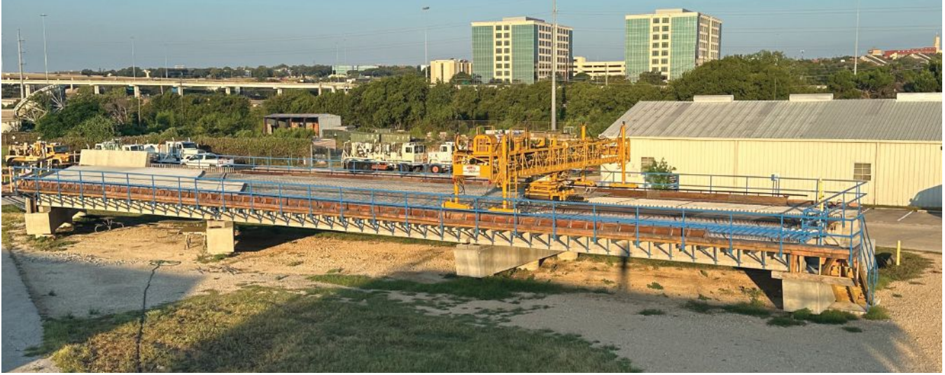
Specimen for the Bridge Deck Construction Inspection Training Facility. Photo: Concrete Bridge Engineering Institute.
