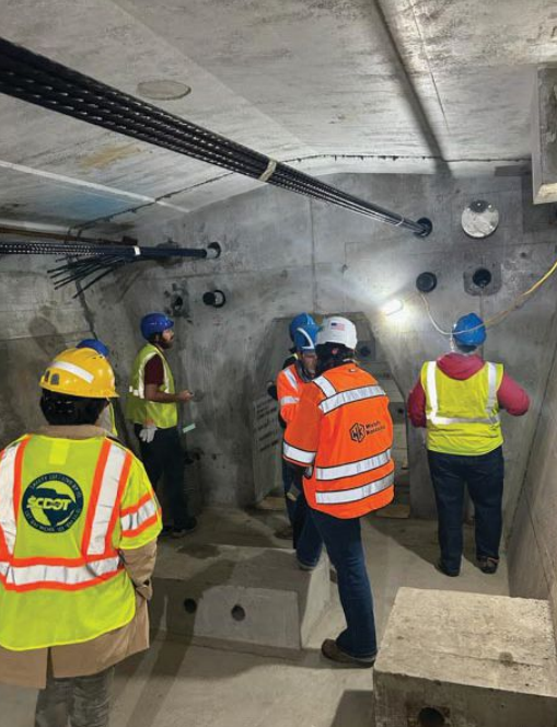
Workshop attendees view the unducted epoxy-coated strand inside the Laurel Fork Bridge. Photo: Jon Cornelius, Sumiden Wire Products Corporation.
