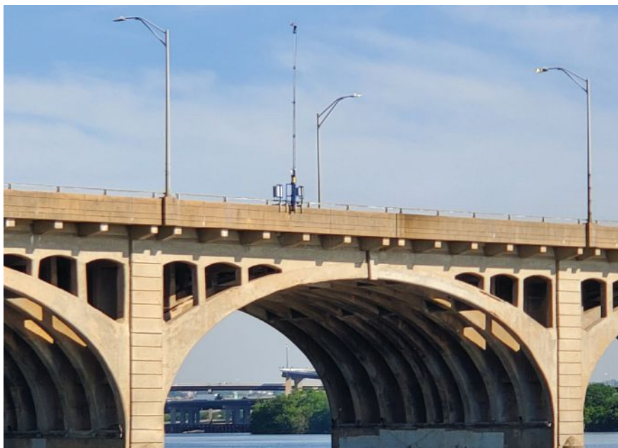
On the Hanover Street Bridge (Vietnam Veterans Memorial Bridge) in Baltimore, Md., infrared ultra-time domain measurements were taken to assess subsurface defects in the concrete deck. All Photos: Fuchs Consulting Inc.
