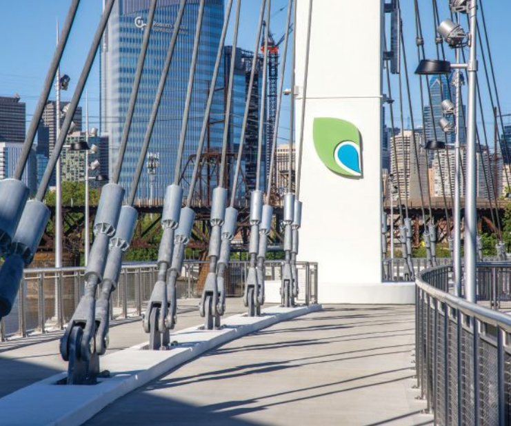
The center-cable arrangement with streamlined pin-and-clevis cable anchors supports the superstructure. Photo: Michael Worthington, Jr.; Worthington Images.
