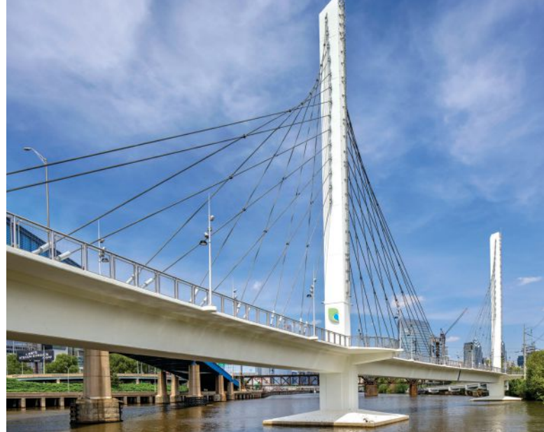
The bridge features a streamlined, curved precast concrete spliced U-beam superstructure with cables in a basketweave pattern. Photo: Michael Worthington, Jr.; Worthington Images.
