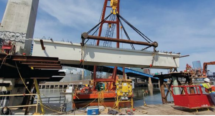
A barge-mounted marine salvage crane with a crawler assist crane is used to lift the U-beam segments onto temporary falsework. Photo: Pennsylvania Department of Transportation.
