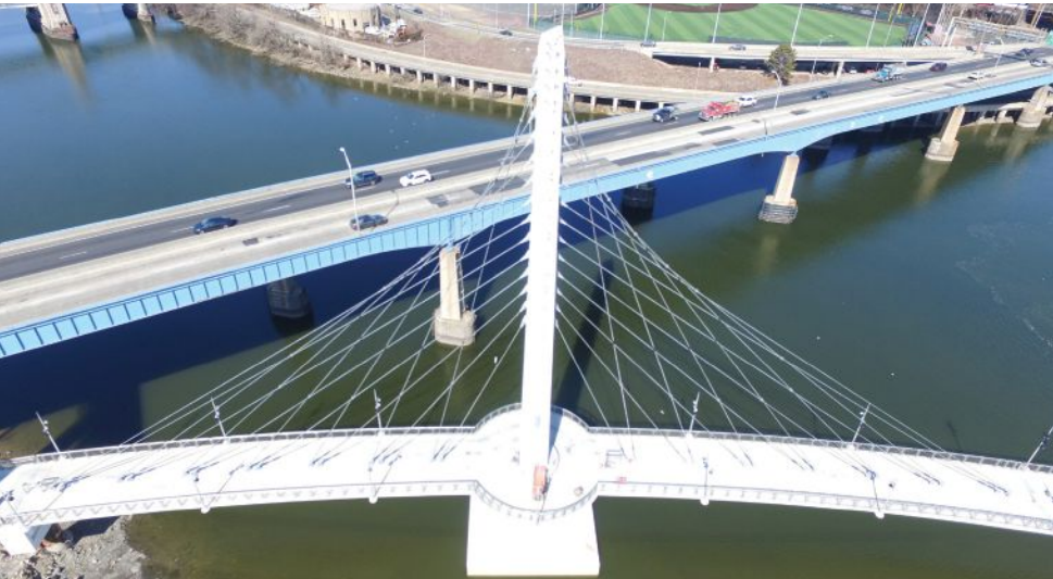
View of the basketweave pattern of the center stay cables shortly after the cables were tensioned. Photo: Pennsylvania Department of Transportation.
