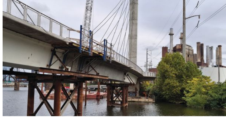
U-beam segments sit on temporary falsework after the deck is placed but before cables are tensioned. Photo: AECOM.
