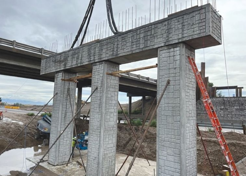
Precast concrete columns and pier caps receive the same rustic quarry stone pattern used throughout the Fort Hall interchange project near Blackfoot, Idaho.
