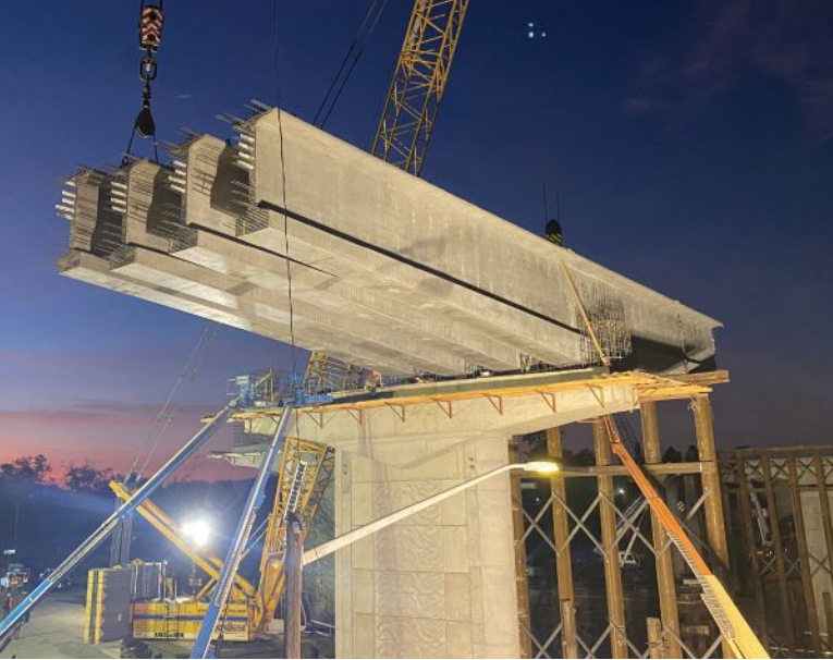
Erection of the haunched girder segments. Photo: Knife River Prestress.
